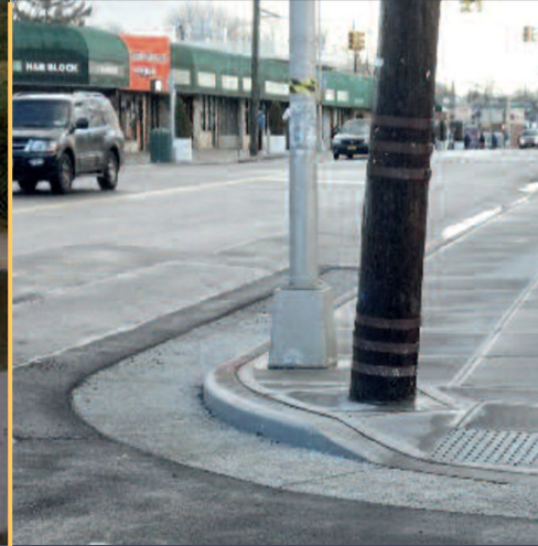
Stormcrete after a 1.5" rainfall
