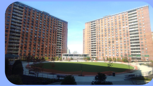
External central circular courtyard
